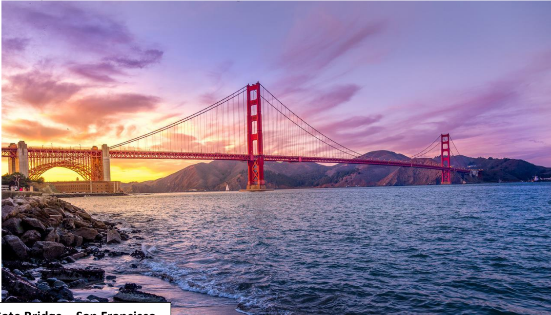
Golden Gate Bridge – San Francisco
